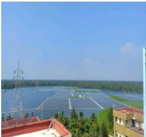
Photo 4: Solar Floating Power Plant
